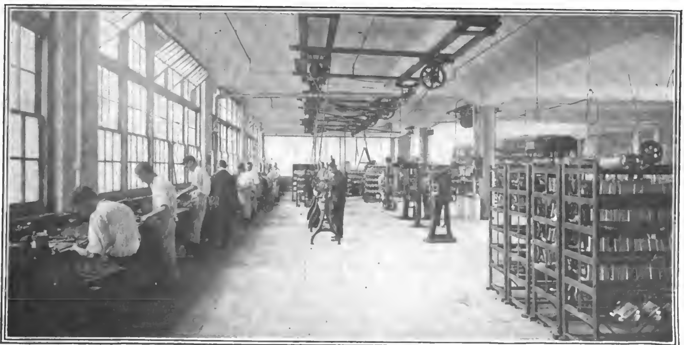
Machine toolroom and assembling floor of the factory, showing a general scene in the interior of this important section of the new plant. Light is plentiful and space has been arranged with a view to efficiency
